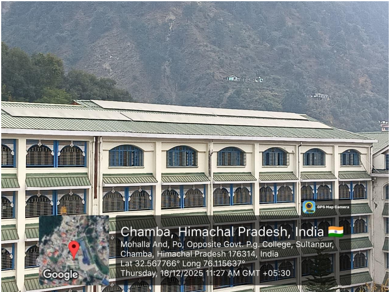
Image: Solar panel installation on the rooftop of old building
