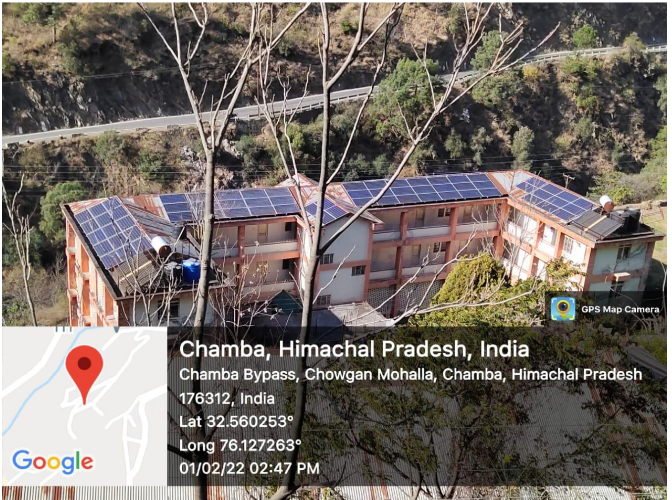
Image: Solar panel installation on the rooftop of Hostel building
